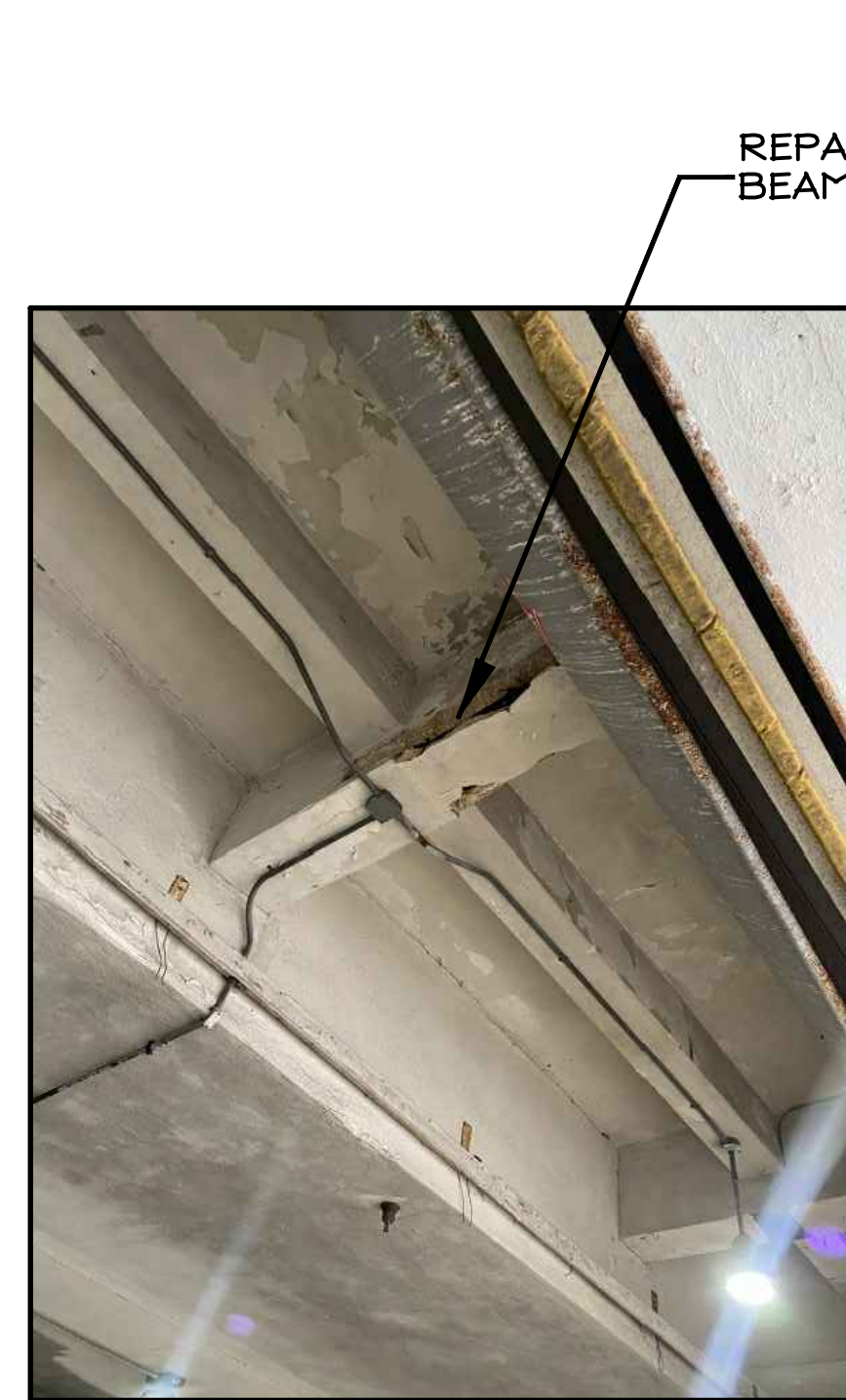
REPAIR TYPE "I" BEAM (TYPICAL)
