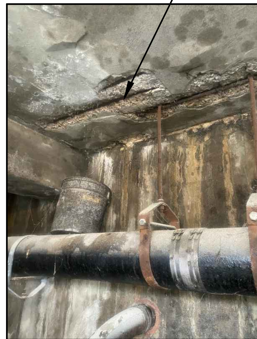
REPAIR TYPE "J" SPALL (TYPICAL)
