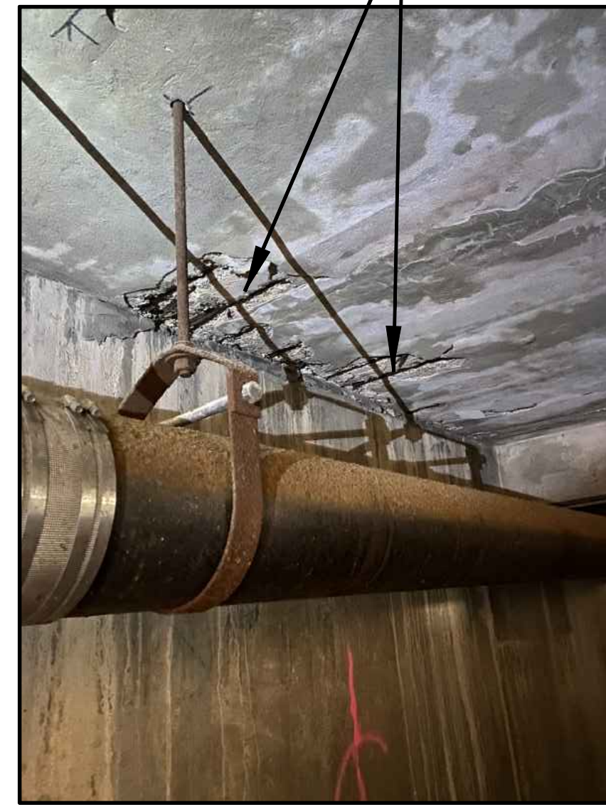
REPAIR TYPE "J" SPALL (TYPICAL)
