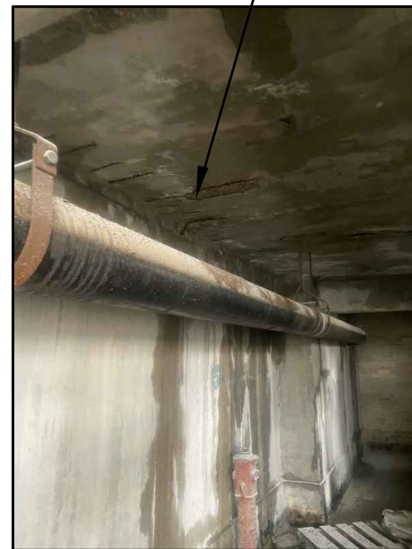
REPAIR TYPE "J" SPALL (TYPICAL)
