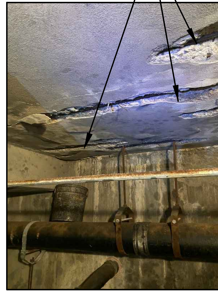
REPAIR TYPE "J" SPALL (TYPICAL)
