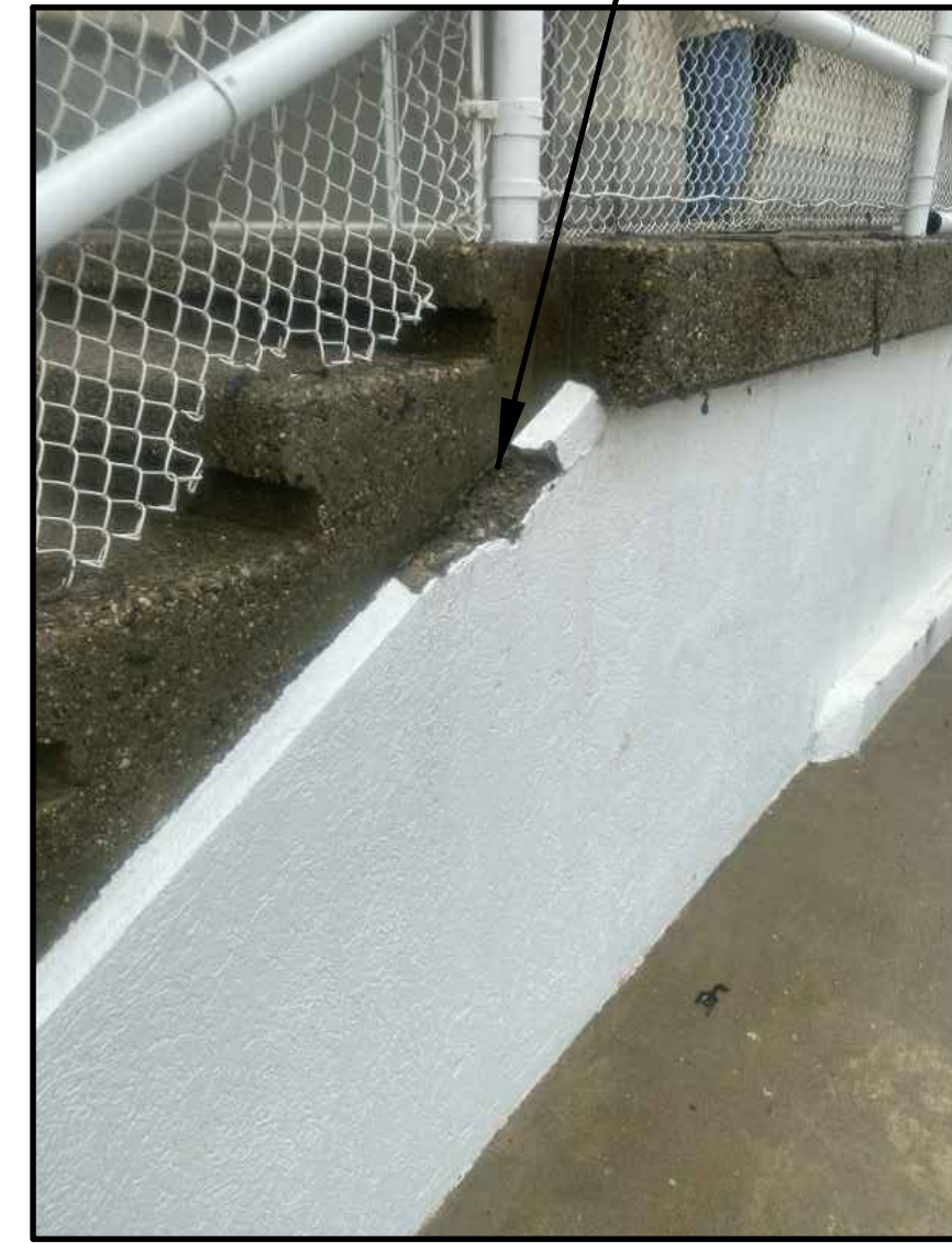
REPAIR TYPE "H" PATCH (TYPICAL)
