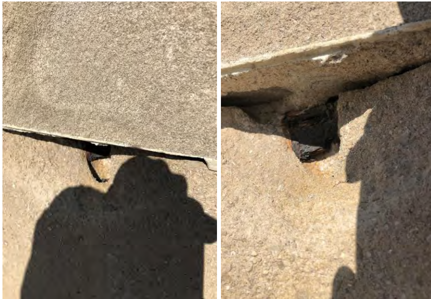
Fig 4: Left: Corroded anchor set in Lewis (Lifting hole) / Right: Close up view of corroded anchor
