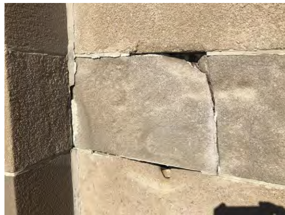
FIGURE 5C: SIGNIFICANT DAMAGE TO STONE IN FRONT OF SPANDREL BEAM
