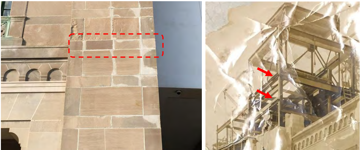
Fig 8: Left: Significant repairs and also cracking through thinner stone course below the shelf angle confirms active corrosion to the steel (See also Appendix Figure 2 for likely angle position in stone) / Right: Historic construction photograph (provided by PFA) revealing existence of shelf angles attached to spandrel beams
