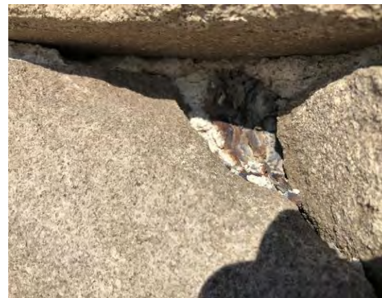
FIGURE 5D: CLOSE UP OF CORRODED ANCHOR – COVER DEPTH 1½"
